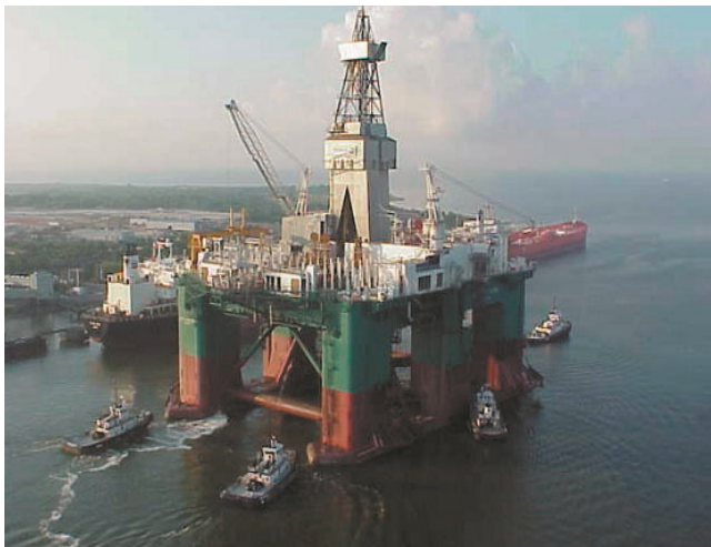
Crane safety and drill string
